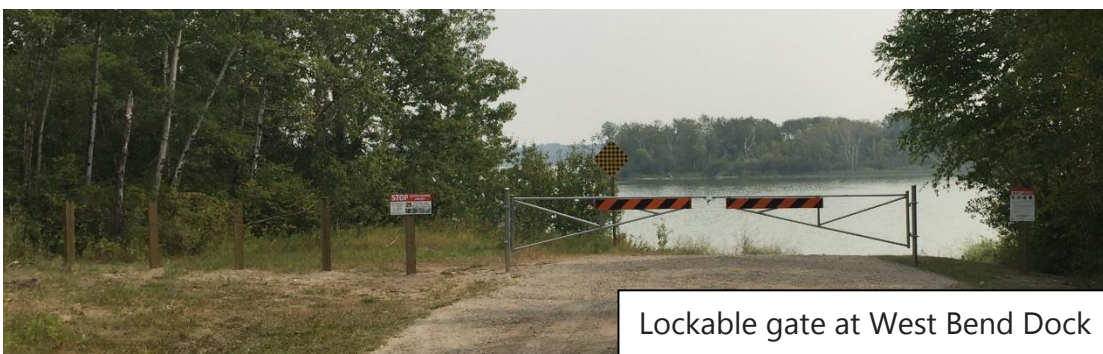
Lockable gate at West Bend Dock
